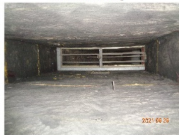
Lined Ductwork After Cleaning
